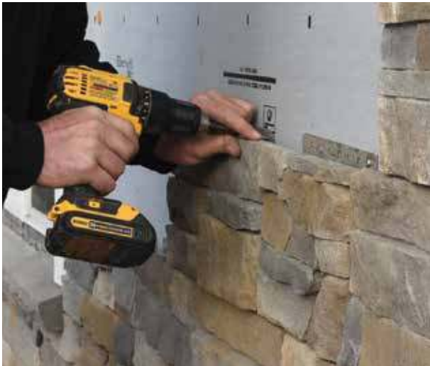
Easy-to-install stone veneer panels.
